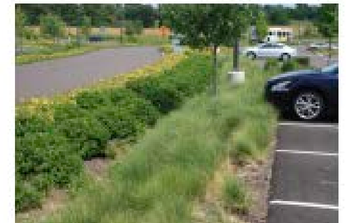
Infiltration trenches at Einstein Hospital in East Norriton. Photo Credit: Montgomery County Planning Commission/Plickr CC
