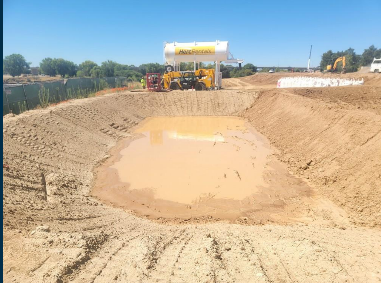
PHOTO; BENTONITE SLURRY DEWATERING; LEVEE CUT OFF WALL PROJECT
